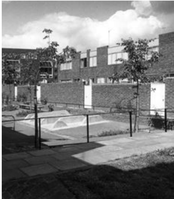
Figure 14: View of a play area (1975)
