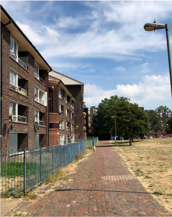
Figure 31: Park edge formed by existing buildings to north east
