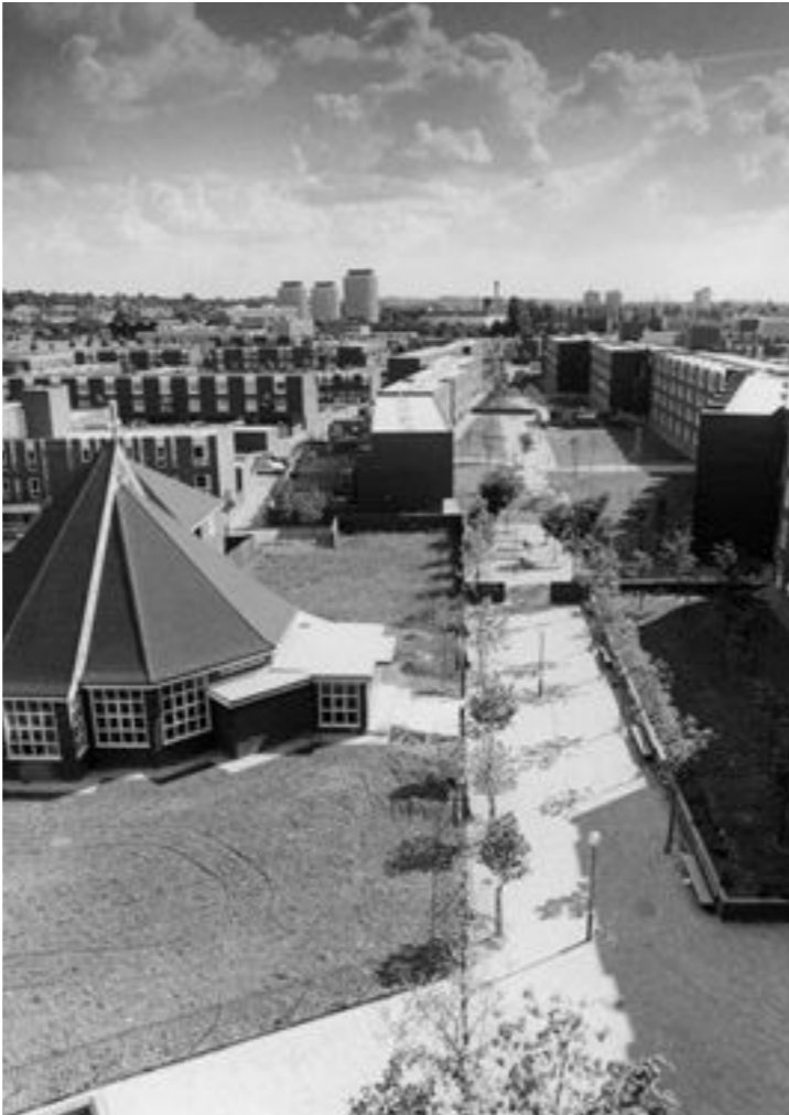
Figure 9: View of St Augustine's and the northern concourse (1975)
