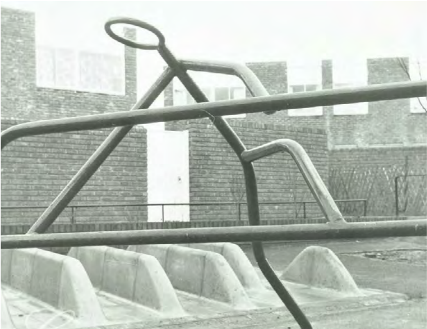
Figure 13: Tubular steel and concrete play equipment (1973)
