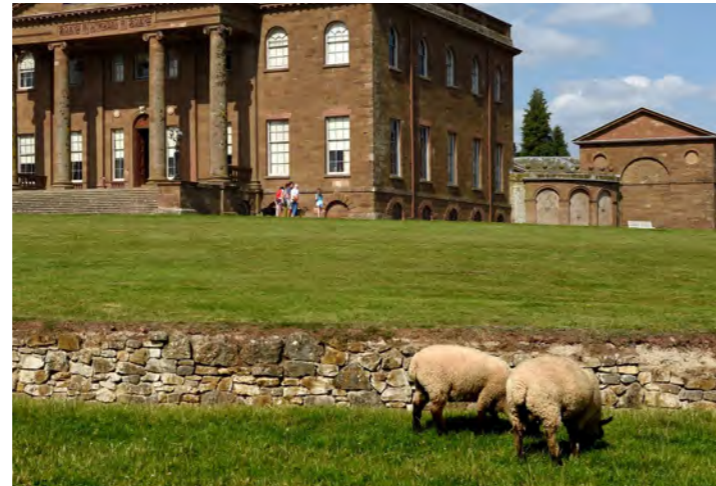
Figure 95: Traditional sunken Ha ha creates a seamless, invisible threshold between arable land and lawns when viewed from the gardens.
