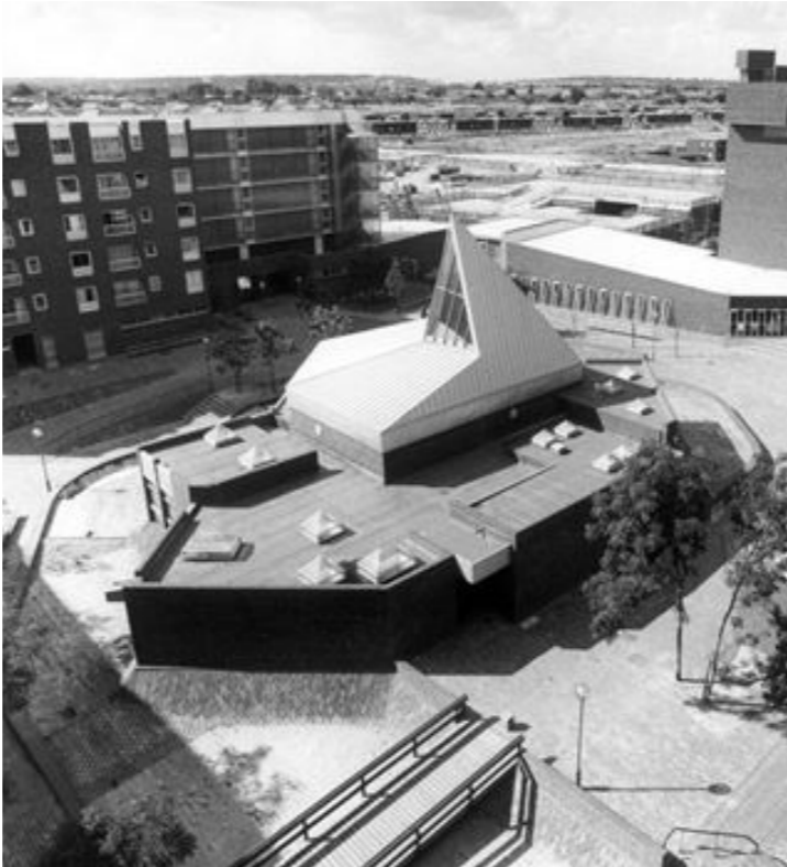
Figure 10: View of the dry moat to the Community Centre (1975)
