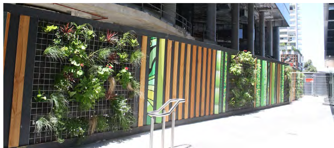
Figure 150: Landscape reducing the impact of temporary hoarding
