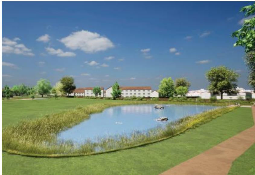
Figure 6-4 Design visualisation of the proposed SuDS basin filled post heavy rainfall Image Credit: Barnet Council
