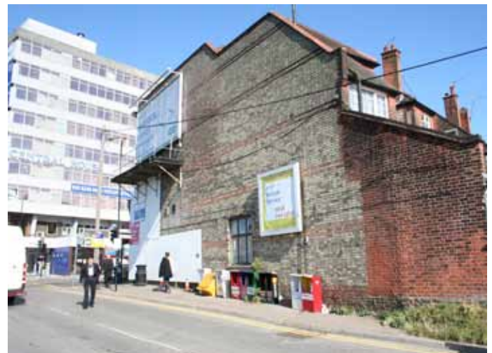
Poor advertising and signage
