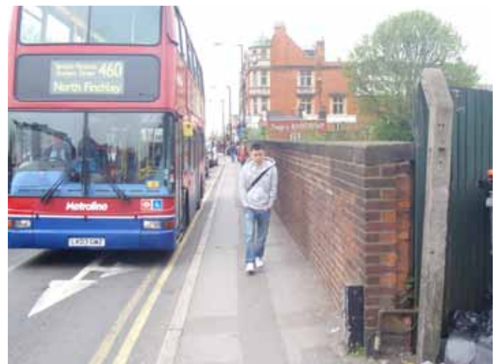
The bridge over the railway lines
