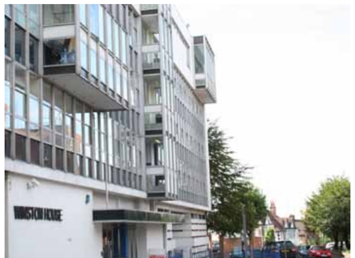
Office space at Winston House
