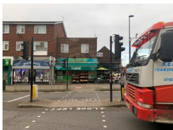
Lack of pedestrian crossing phase at signalised junction
