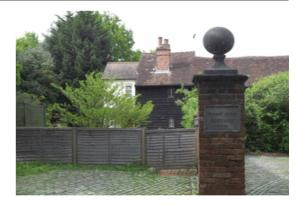
**Description:** Two storey house in dark weatherboarding and render with clay tile roof and brick chimney stacks. Small window openings with sliding sashes. Evidence of sagging to roof structure. Retains original features and character.
