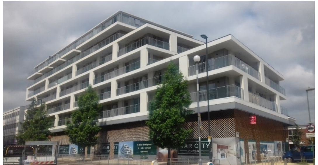
23 – Greenpoint, Edgware Road
